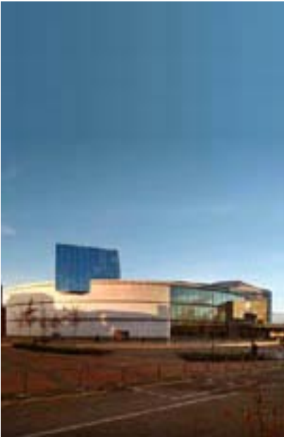
The Helix Centre, Dublin
